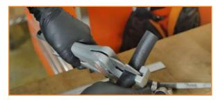
14. Combine the two shorter hoses using the 90° fitting to make your outlet hose.(2x worm gear clamps)
