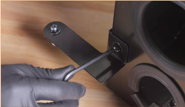
05. Install one of the supplied mounting studs to the bottom of the long bracket. Leave the bolt loose for now. (1x 4mm Allen bolt, 1x lock washer, 1x metal washer)
