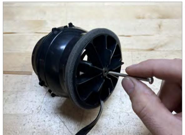
**6** Insert #6 2 inch screw (provided) into hole in back of vent housing
